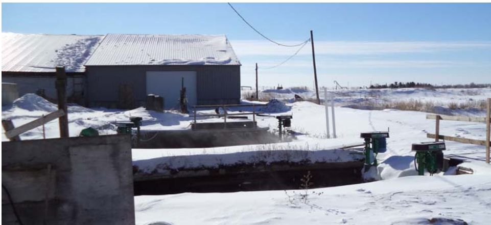
Photo 2 – Central collection pit and agitator to mix manure from barns
