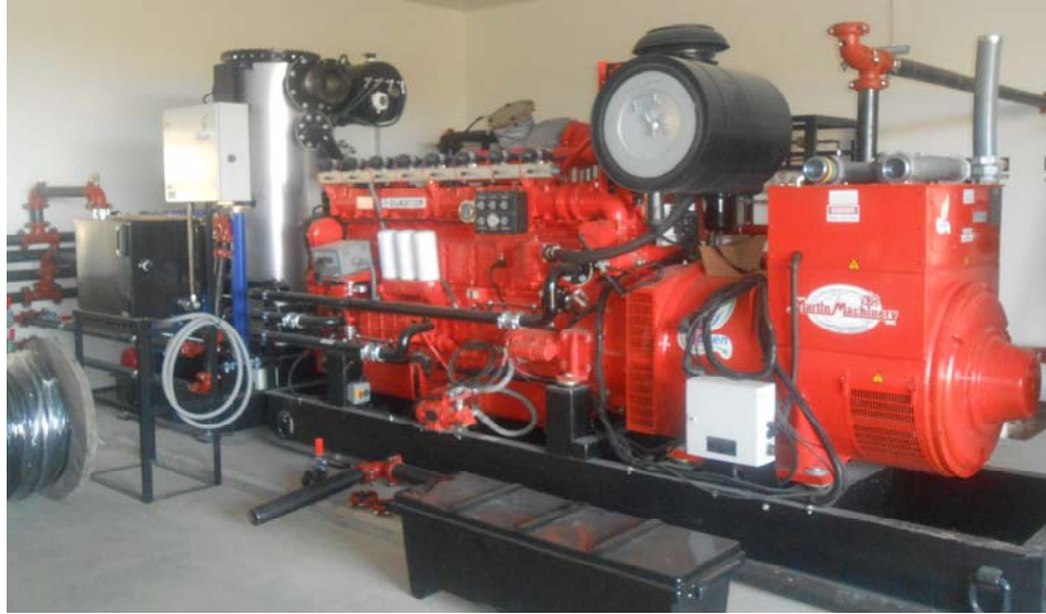
Photo 6: Engine and 300 kW generator
